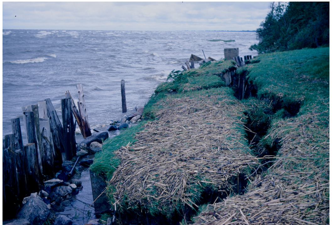
Figure 38. The bank adjacent to Mallard Lodge after strong winds from the north had caused considerable erosion, summer, 1971. Note the remains of the palisade on the beach.
