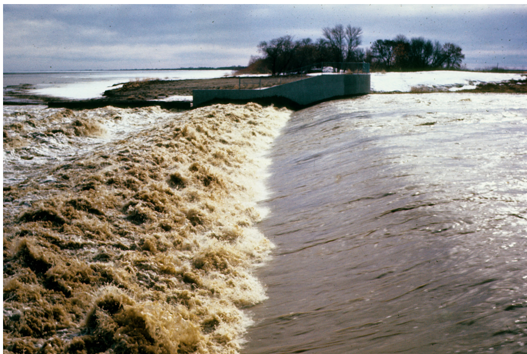
Figure 33. The Portage Diversion in action for the first time. Water flowing over the Diversion outlet sill into Lake Manitoba, spring 1970.
