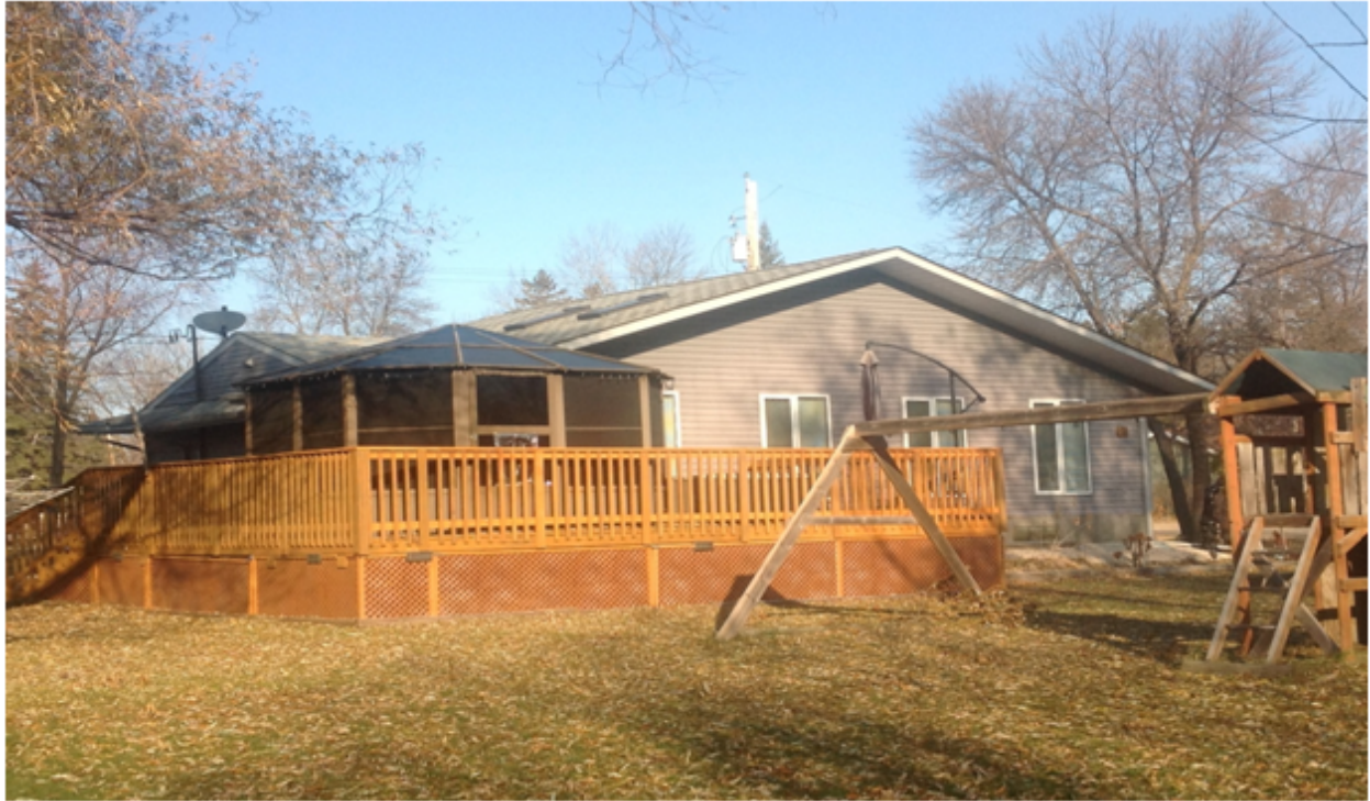
The renovated cottage as it stands today
