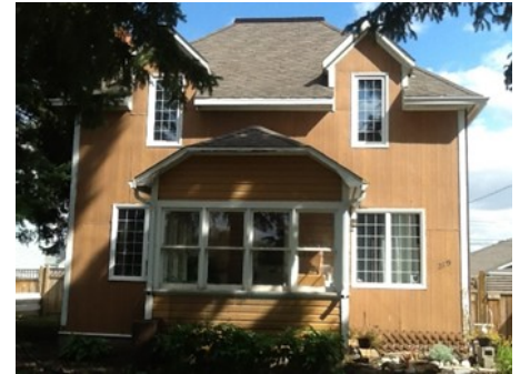
219-5 th Ave. N Built in 1905 by William McKenzie and Donald Mann, owners of two small railway companies which amalgamated to form Canadian Northern Railway. One of these small companies, The Winnipeg Great Northern continued building railways from Sef-ton to Swan River Valley. It is likely this home may have been built for one of their workers. The Norman Garland Family lived there for many years. The inside has been changed extensively.
