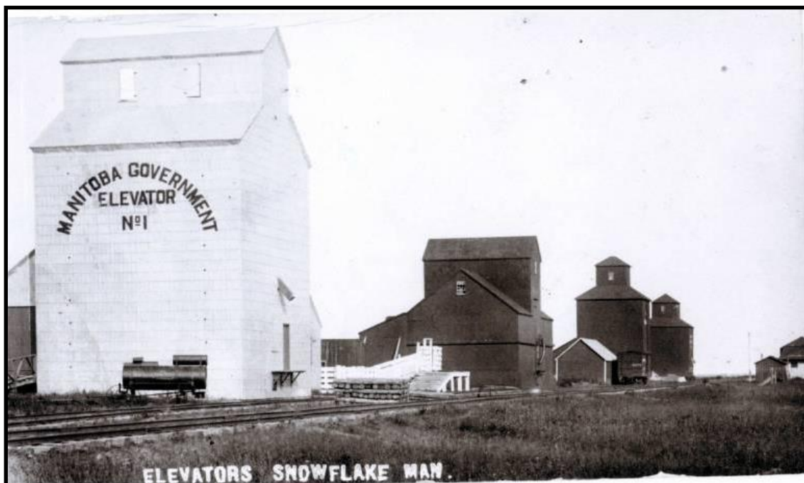
Figure 10: Snowflake Elevator Row, circa 1910. Left to right: the Farmers' Elevator (built in 1904); livestock corral and loading dock; the Canadian Elevator (originally a warehouse built in 1902); a coal storage shed; the State Elevator (built in 1900); and, at the western end of the line, the Imperial Elevator (1901). Partially visible at the far right is the CPR stationhouse and freight shed. By the 1930s all but the Farmers' Elevator had been demolished. In 1928 a Manitoba Pool Elevator was constructed on the former site of the Canadian Elevator, and in 1962, Snowflake's last elevator, the Federal Grain Elevator, was constructed on the former site of the old State Elevator.
