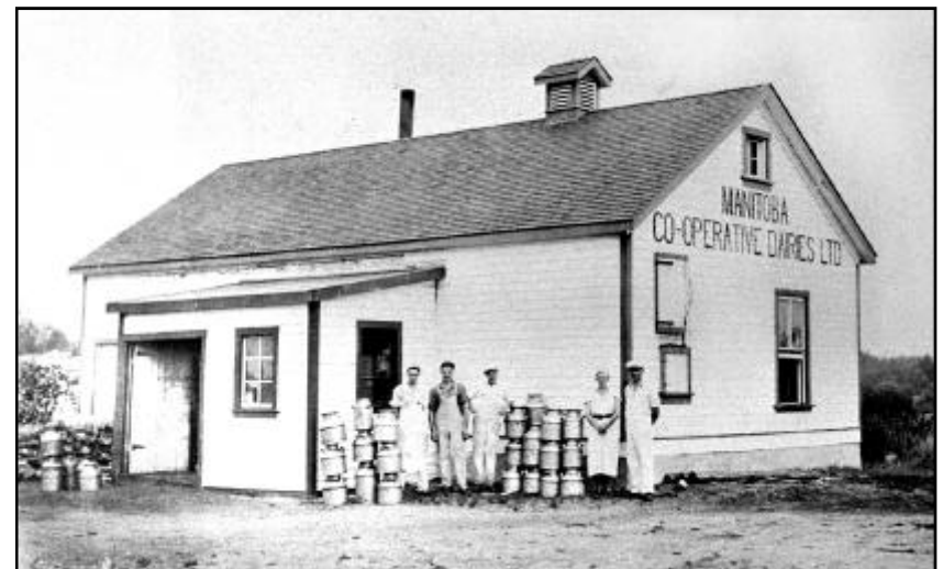
Above: Chatfield Creamery, 1936. Constructed in 1933-34 by Manitoba Co-op, it was managed by Harry Hawkins for the first seven years. Later owners were Mr. Anderson and John Yaremy who operated from 1942 to 1976. NC,CH-008.
