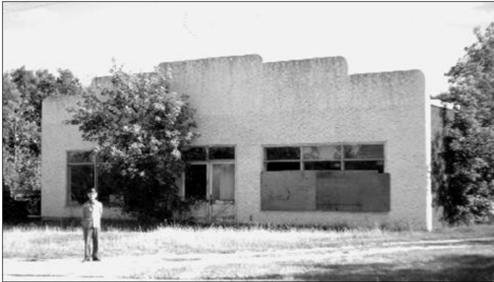
Above: Mike Torbiak garage in the old town site, visited by Nick Lisowecki, its builder, in 1974. Mr. Torbiak gave instructions that there were to be no supporting posts in the front showcase and counter area. It was the largest free-span attempted by Mr. Lisowecki and, after completion, was inspected and easily passed by a structural engineer. CL-131.
