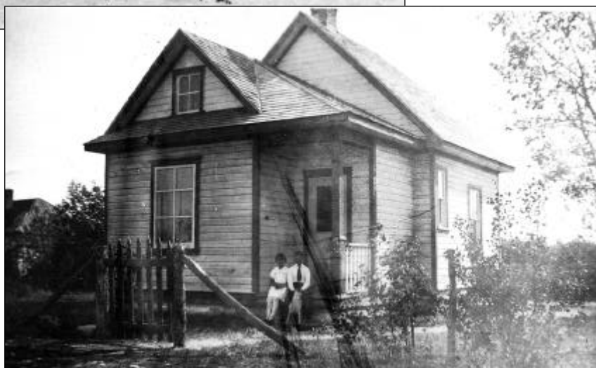
Left: The Nykola Lisowecki house located at the west end of the town, on the south side. Mr. Lisowecki was one of the main carpenters in the Poplarfield district, and constructed many of its schools, churches, stores and homes. He, and wife Justine, raised a family of five girls and a son, and kept a small dairy herd for extra income. This photo was taken during the early-1930s. Sitting on the front steps are Olga and Peter Lisowecki, and 'Skipper'. CL-005.
