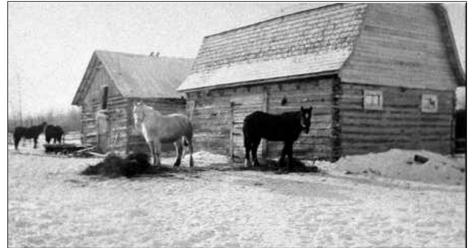
Above: Log barns on the Peter and Katherine Ledochowski's Hamrlik P.D. homestead. Structures of this type were typical of the first permanent set of farm buildings constructed by the pioneer families. FL-130.
