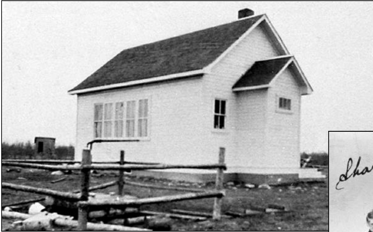
Left: Sharpewood School No.1867, c1935. Sharpewood School was constructed in 1918 on SW 16-22-3W ten miles west of Poplarfield. SC,SH-001.
