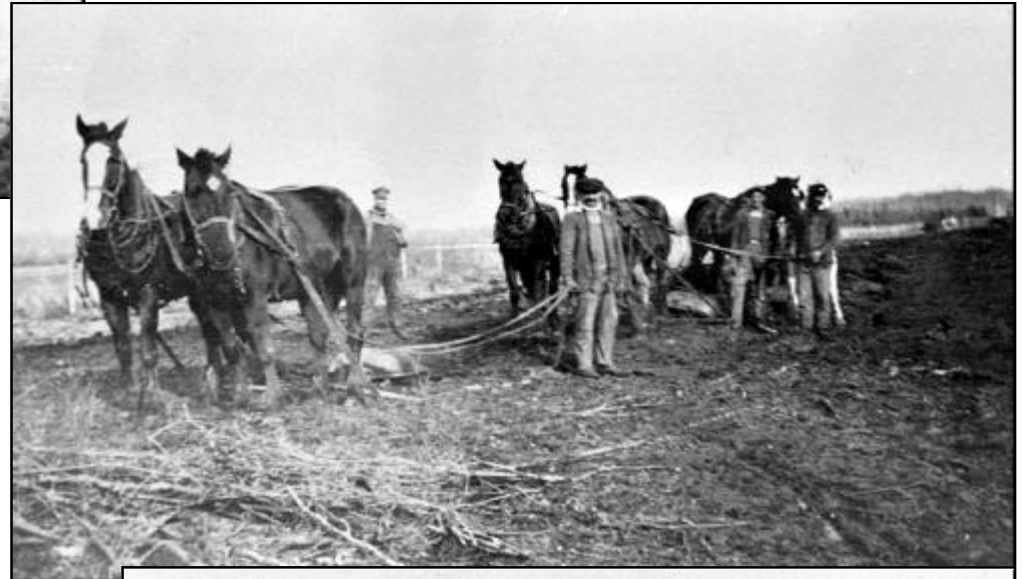
Left: Road construction in the Chatfield area, using teams of horses and hand-held scrapers, c1935. Prior to this period of road construction during the Great Depression, most roadways in the region were simple trails, level to the ground and very rough, making motor vehicle travel slow and difficult. The first raised and graded Provincial Roads were constructed with the 'statute labor' programs of the 1930s and provided the district with its first few proper roads. Truck transportation very quickly became commonplace once the road system began to develop. RTM-021.
