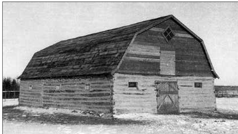
Above: Typical log barn of the 1920s and 1930s era, this one is the original Swarychewski barn, now possessing a North American style 'gambrel' roof. FL-092.
