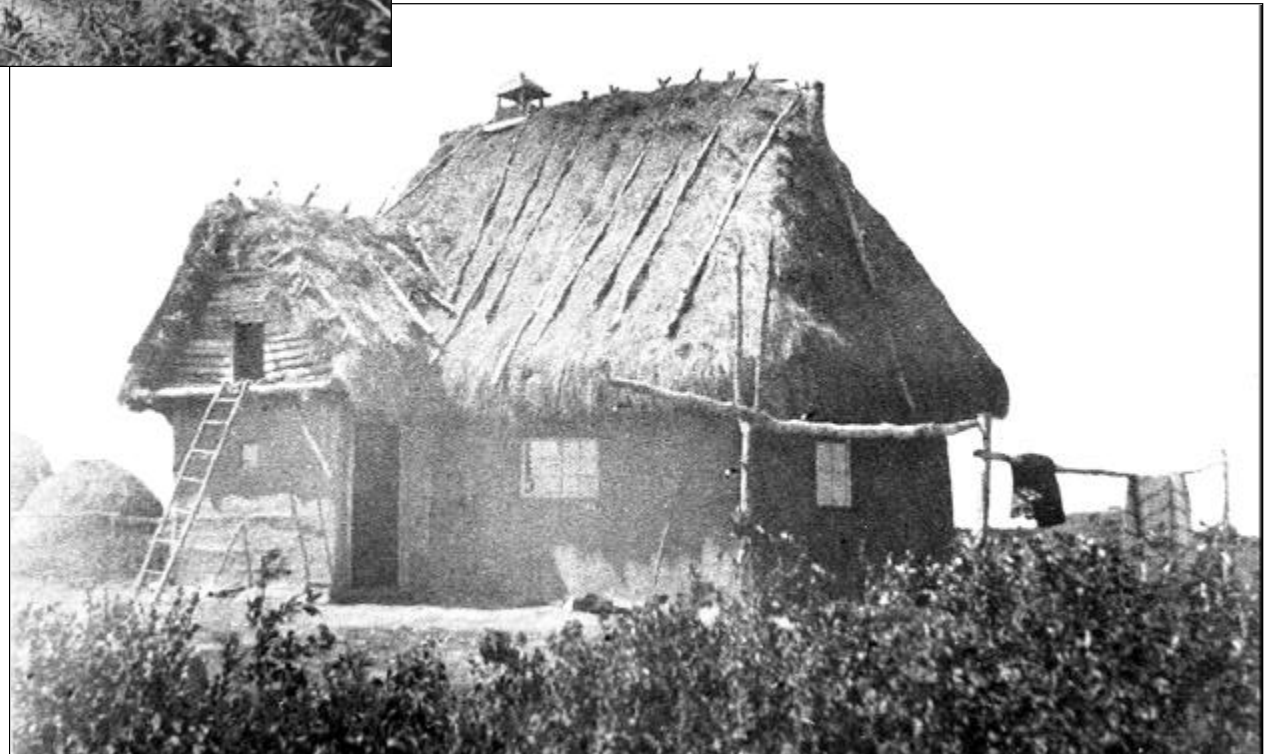
Right: Photograph of a typical first home constructed by Ukrainian settlers in Manitoba. Usually quickly and roughly built, such initial structures were not meant to last more than a few years. Most were made in one summer using a few simple hand tools, a handful of hardware, and a few panes of glass. Among other things, this interesting little home exhibits: a roof of loose hay held in place by criss-crossed poles; home made boards used in making the gable front over the entranceway, permitting access to the attic; and a thick, smooth coating of mud plaster mixture. Note also the poles being used as a clothesline, and the home-made ladder. PE-002.
