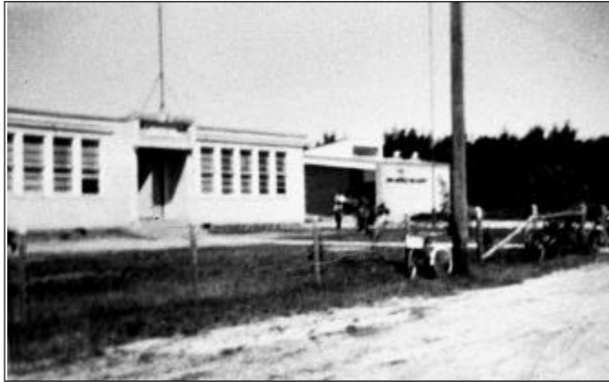
Above: View of the third Dehowa School, constructed c1954, and the Poplarfield Collegiate building, constructed 1962, in the background. SC,DE-034.
