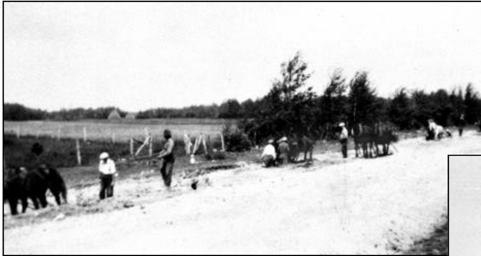
Right: Another view of a road construction crew at work building up a roadway using only horses and scrapers, 1930s. RTM-029.
