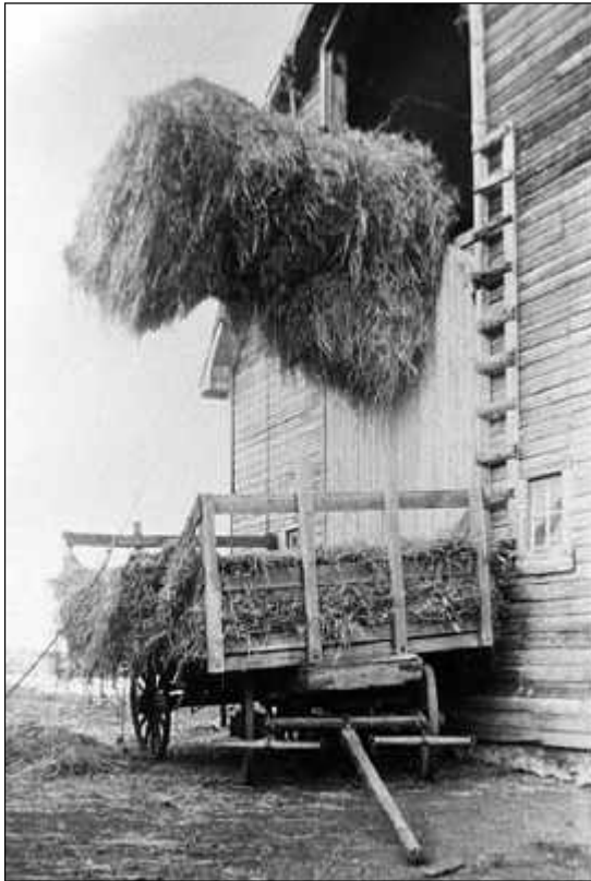
Left: A hay-sling in action. The hay sling was fitted on a few of the larger barns in the district. The cable and pulley mechanism was a great labour saving device if you could afford one. FL-075.
