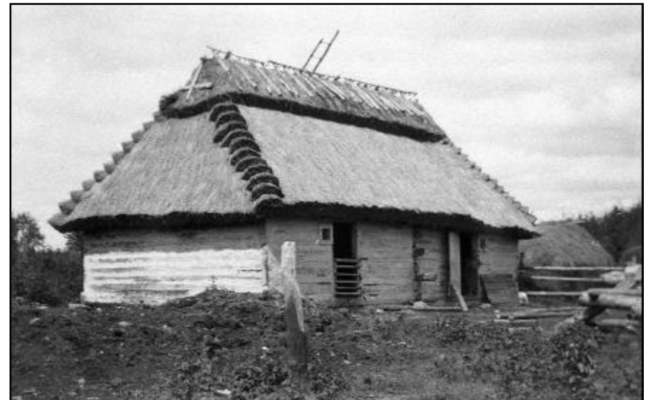
Above and lower left: Good examples of well-crafted 'old country style' farm yard structures. Note the superb job of thatching, on both structures, and the nice straight walls and plaster finish on the two-roomed barn. Clearly, skill, time and effort went into the construction of these pioneer farmyard buildings, suggesting how important the livestock was to the early settlers. PE-019, PE-035.
