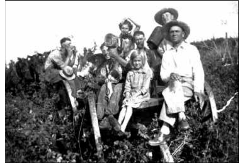
Above: Stopping for a lunch break while piling roots and stones on the John Sotious farm, New Star District, 1938. The many low ridges in the district were full of stone, which had to be picked not only during land breaking, but almost every year due to frost action pushing the stones to the surface. FL-015.
