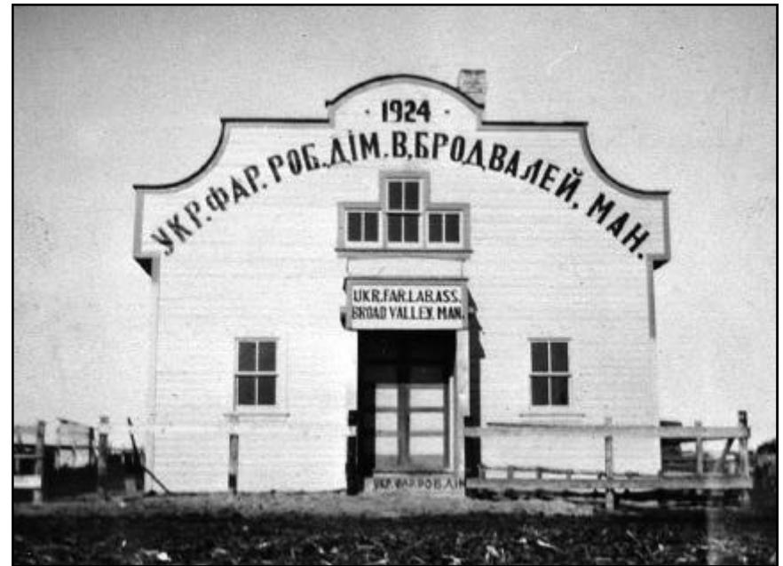
Above: The "Broad Valley Ukrainian Farm Labour Association" Hall, constructed 1924. NC,BV-004.
