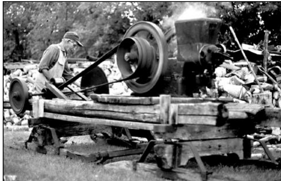
Bill Pawluk sawing firewood with a one-cylinder stationary engine, by himself. Sawing firewood with a rip-saw is a difficult and dangerous job for one person. Here Bill, at 68 years of age, has managed to rip a large pile of firewood without assistance, as winter fuel for his little retirement house which he shared with brother Andrew. Circa 1973. RTM-038 to RTM-041.
