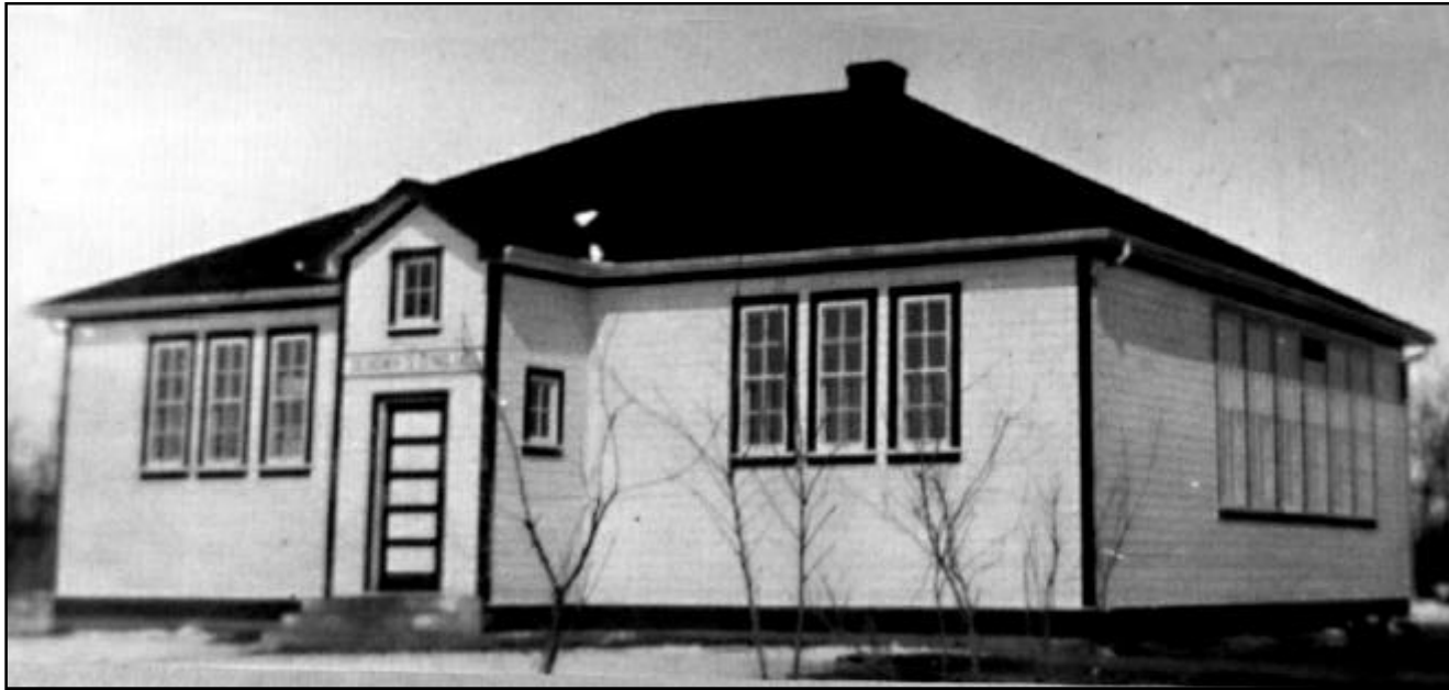
Above: The first Dehowa School was destroyed by fire the winter 1935-36. It occurred in the night as a result of a faulty stove pipe. By the beginning of the next school year a new building was erected in a different location within the school yard; and pictured above soon after its completion. Note the recently planted row of trees. This, and several other rows of trees, grew rapidly and before long completely obscured the public view of the building. SC,DE-043.
