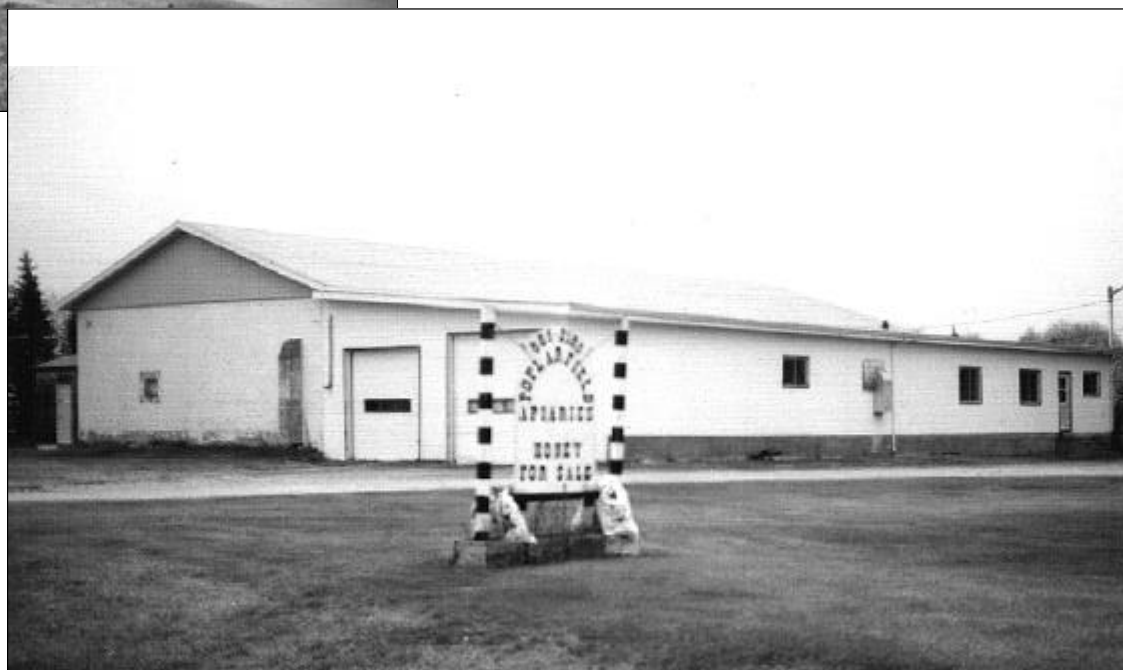
Above and right: The Poplarfield Apiaries, photographed in the autumn of 2000. The structure was originally constructed as the Poplarfield Turkey Company processing plant, but only operated for a few years. It was then purchased by Cecil Fast who converted it into a honey processing plant, taking advantage of the many alfalfa crops being grown in the area during the 1970s. It continues to operate as an apiary, with Leonard Heinrichs as the owner-operator. CL-117, CL-118.
