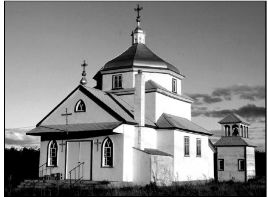
St. Nicholas Church in its new town location, as it appeared during the mid-1970s, now with a covering of white stucco. Note also that the belltower had been enclosed. FR-021.
