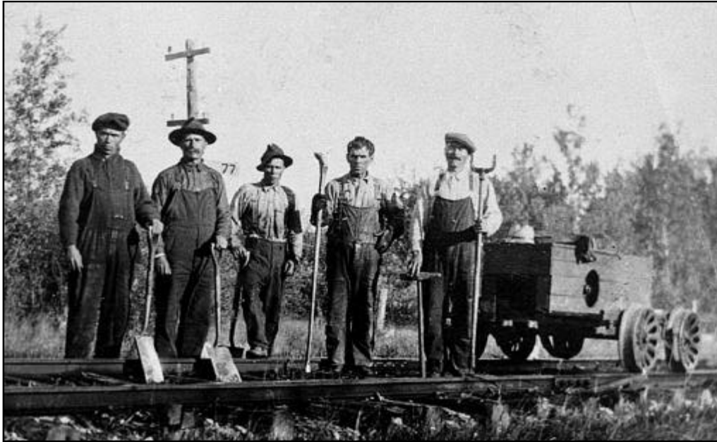
Above: View of a typical 'section gang' doing maintenance work along the right of way, in this case, it is the crew from Hodgson, July 19, 1929. L-R: Bill Mamchuk, Alec Rykunyk, Harry Porcina, unknown, and Mike Stefanec. The Poplarfield Section Gang was known for possessing a very distinctive home made cab on its the motorized "jigger" car used to transport the crews to work sites. RTM-028 .
