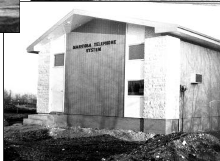
Above: The newly completed Manitoba Telephone System building in 1964. With the installation of automatic switching equipment, the manually operated switchboard first installed in Peter and Luba Bailley's store was removed, and Poplarfield lost its local operator service. Mr. & Mrs Bernie Perras were the last to provide operator service in the Poplarfield exchange district. CL-068.
