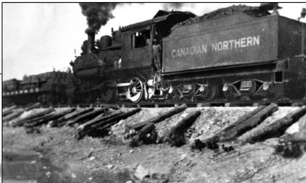
Above: Supply train photographed bringing construction materials to the railhead during construction of the Canadian Northern Inwood Subdivision branchline, 1914. Note that the locomotive is pushing the flatcars to the work site, and also that only every second tie was placed into position during initial construction. Work crews would later fill in the gaps using the ties left along the grade. RTM-002.
