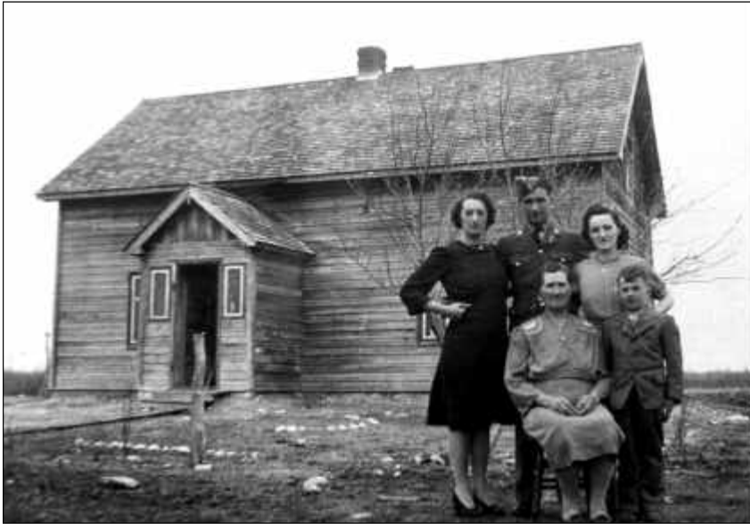
Above: Homestead of Danyla and Natalia Haliuk, located two miles NE of Poplarfield, as it appeared during the 1940s. The house is typical of many homes in the district constructed in the traditional Ukrainian style, upgraded during the 1920s or 1930s with wood siding and wood shingle roof, replacing the thatch roof and mud plastered exterior walls. Natalia seated and daughters Justina and Pearl in rear. FL-078.
