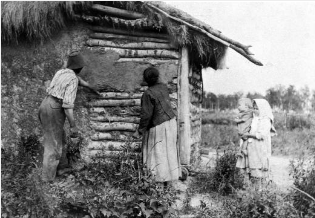
Left: "This house was not as well built as most of them were but it shows the method of construction and particularly plastering with the clay found on the farm. As in many of the districts in the west, there was clay subsoil here. A circular hole about four feet in diameter was dug, the topsoil to a depth of a foot or so was removed and discarded. The clay was then dug and left in loose lumps. Some short straw or hay was scattered on them. Water was then poured over the whole mass, which was next trampled and mixed by the bare feet of men, women and children. The finished product was then applied to the logs by using bare hands as trowels. Such a mud wall would last for some years." - J.W. Sisler, 1906. PE-011.
