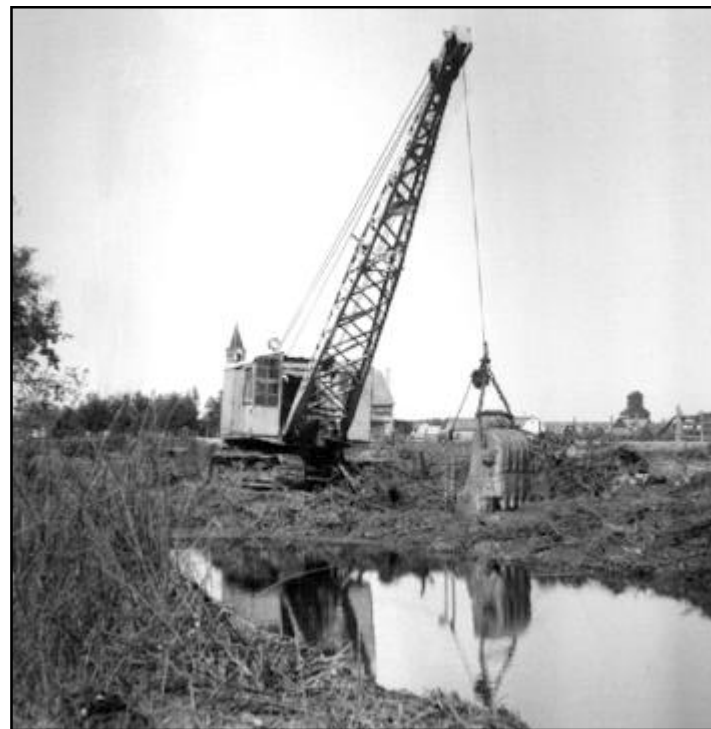
Above: A dragline dredging the Fisher River, to improve the flow and help with the spring runoff, c1940. NC,FB-018.
