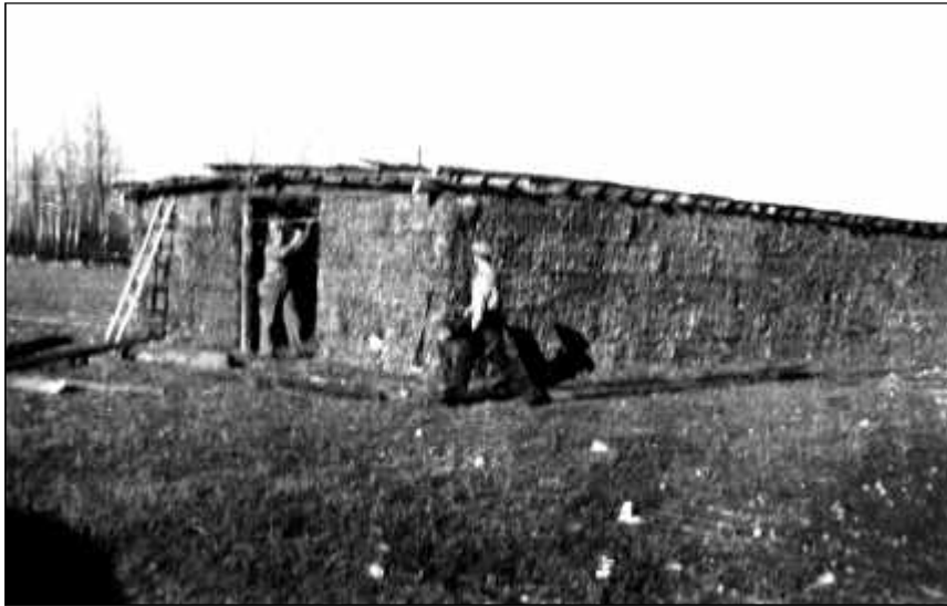
Above: Constructing a sheep barn with straw bales on the farm of Mike Swarychewski, 1940. FL-092.
