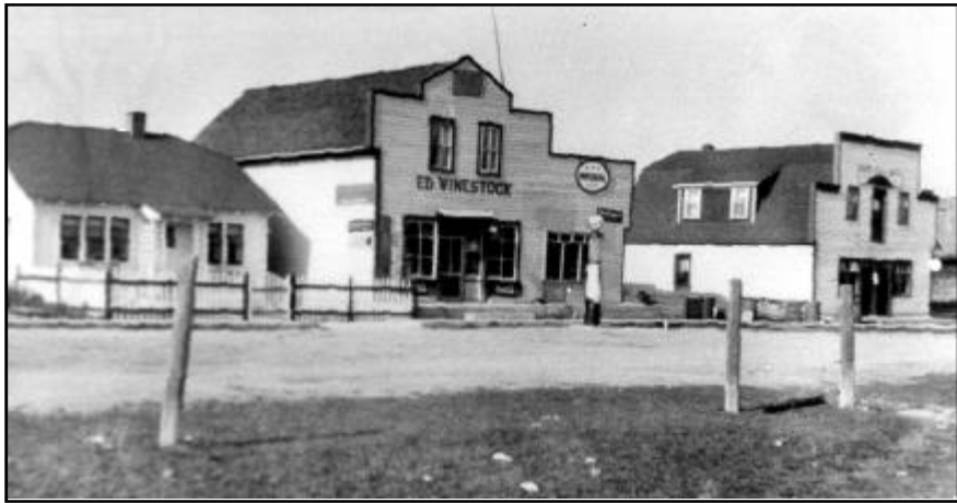
Above: Chatfield, mid-1930s. Winstock's House and Store. Rindall's building intended to be a hotel, used by the Hoborough family as a rooming house. NC,CH-003
