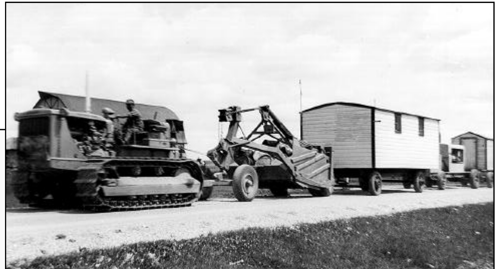
Above and right: On higher ground, during the 1940s the dragline was not required for digging out the ditches for roadbed material. The job was normally done using a caterpillar and large four-wheeled scraper such as the one photographed in operation building up PTH#17 south of Poplarfield on July 7, 1942. RTM-068, RTM-069.
