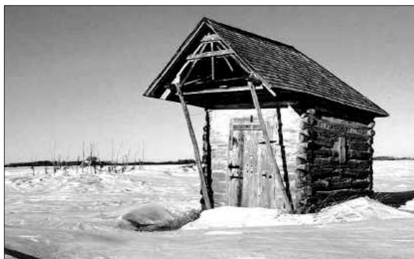
Above: A very well known local landmark. This unusual little shed with its oversized 'hip & gable' roof was located two miles east of Poplarfield along PTH#68. Belonging to Jacob Melynk, it was frequently photographed and survived until 1998. FL-098.
