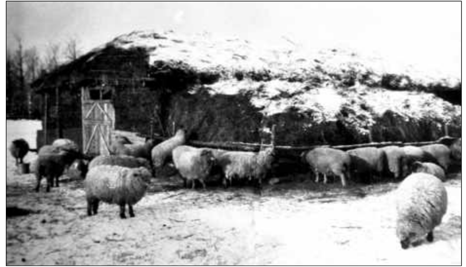
Above: The completed sheep housing building constructed of straw bales and loose hay. FL-066.
