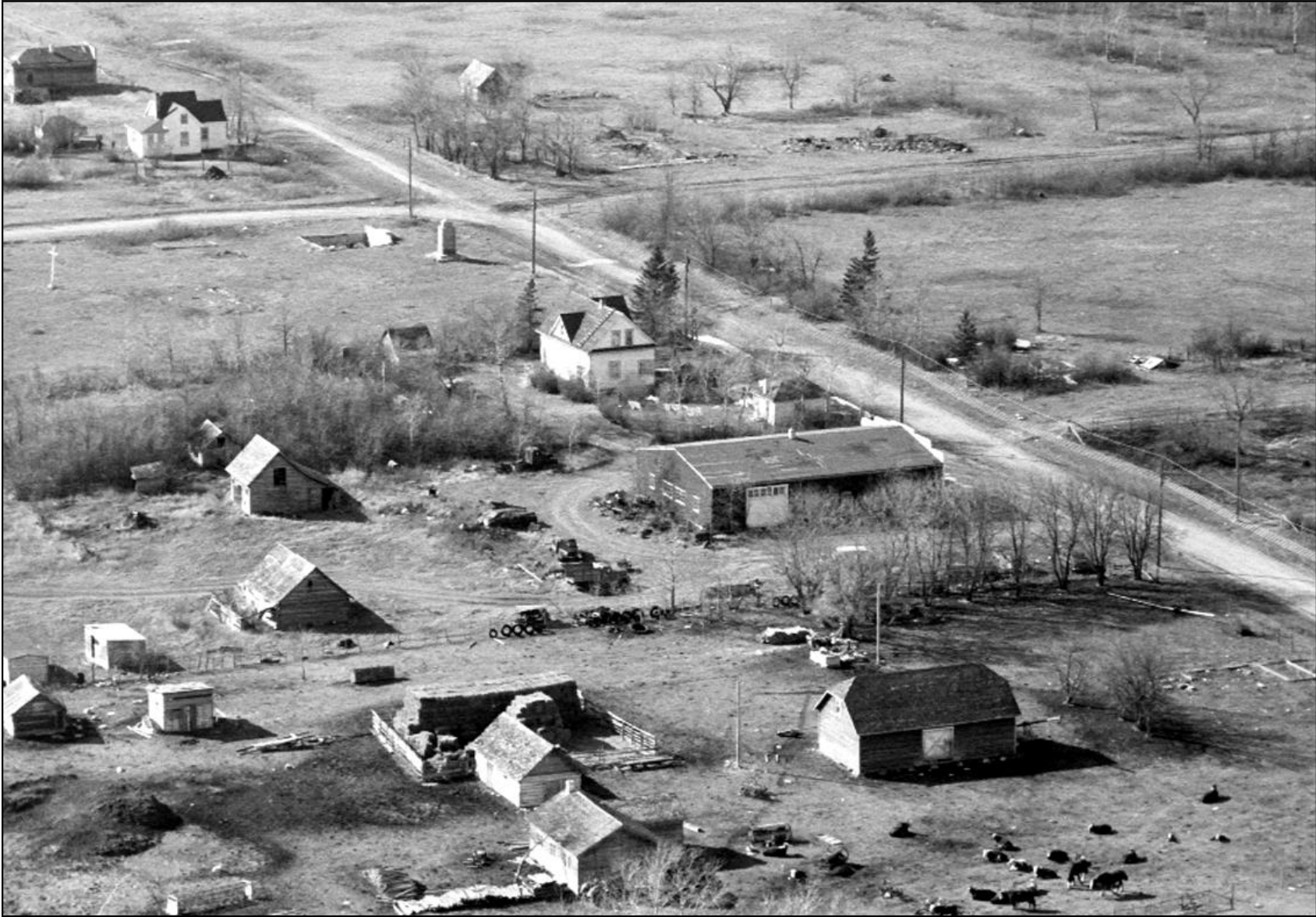
Above: Aerial oblique view of Poplarfield, old townsite, 1973. Besides the surviving structures, eleven other buildings existed at one time within this same view. CL-077.
