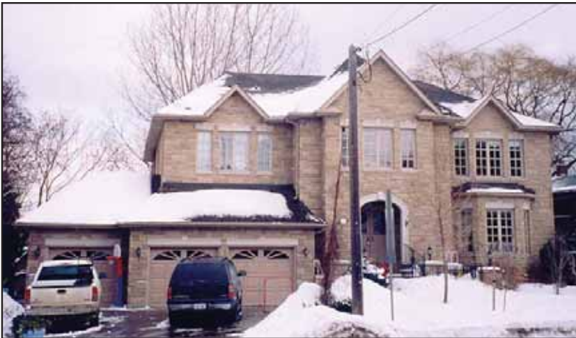
Brian took over the family construction business after Thomas Feeley's passing in 1991, and in 1995 built this home for his wife Mary Jayne. During an average year the company builds about fifty to fifty-five homes in the Toronto area.
