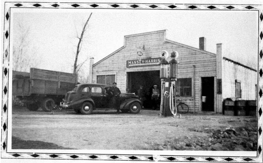
The National Garage in New Poplarfield, built by Stefan's son Mike in the fall of 1939. The Garage was also used for storing freight associated with the Transfer Business which Mike and brother Walter also established at the time.
