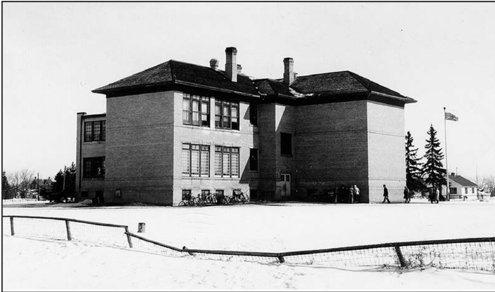
Above. A photograph taken from the west side of the school grounds showing, at left, part of the two storey, two classroom addition constructed in 1941 in the northwest corner of the building. ( Heritage Classroom Coll. )
