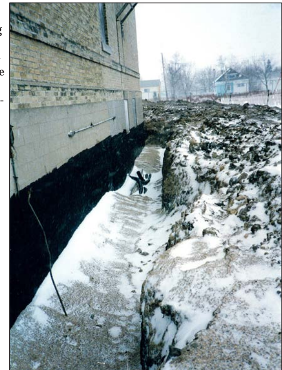
Above and right. Views of the excavations involved with installing weeping tile drainage around the perimeter of the building and applying a tar exterior coating to the basement walls. Another major undertaking for the heritage committee. ( Heritage Classroom Coll. )
