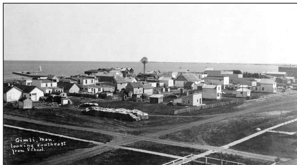
Above. A photograph taken same time and vantage point as the previous, this time looking south east, towards the town centre and harbour area. The windmill in the centre of the photos was built by the CPR to pump lake water to the water tower located near the station on Seventh Avenue. Note the rows of neatly piled firewood. (Gimli Saga Manuscript, 1973 Pg. 566.)
