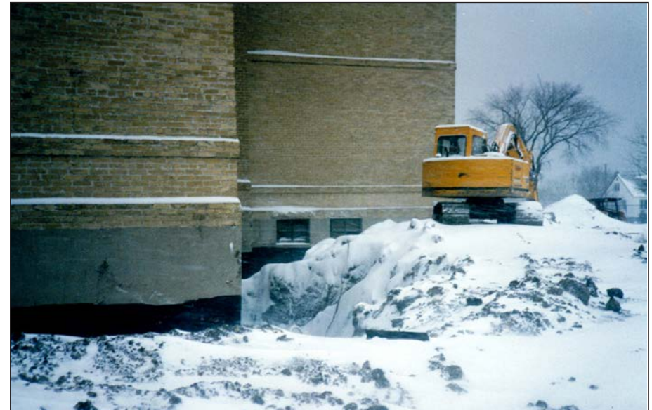
Above and right. Views of the excavations involved with installing weeping tile drainage around the perimeter of the building and applying a tar exterior coating to the basement walls. Another major undertaking for the heritage committee. ( Heritage Classroom Coll. )
