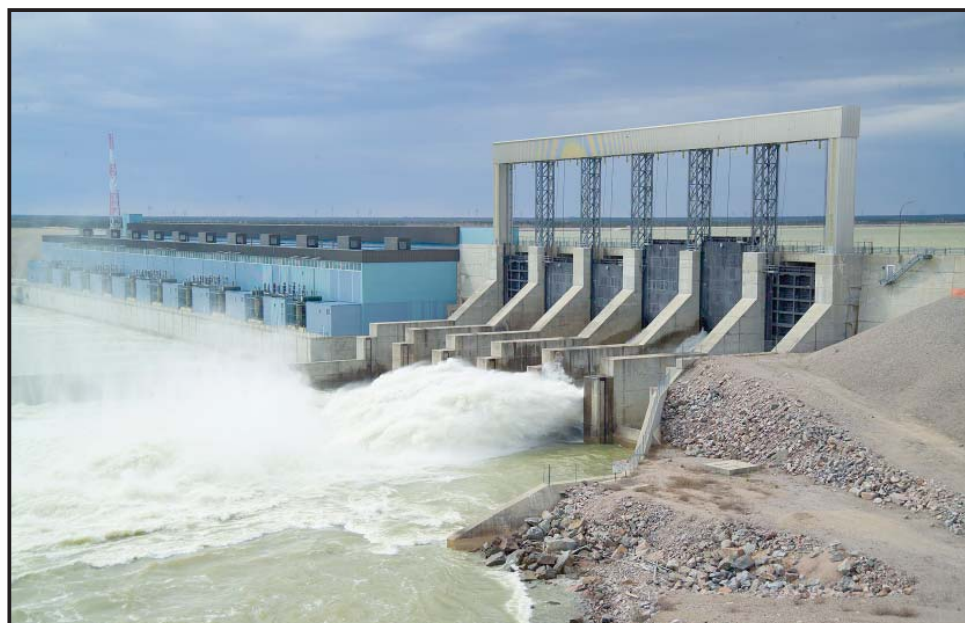
Long Spruce spillway.
