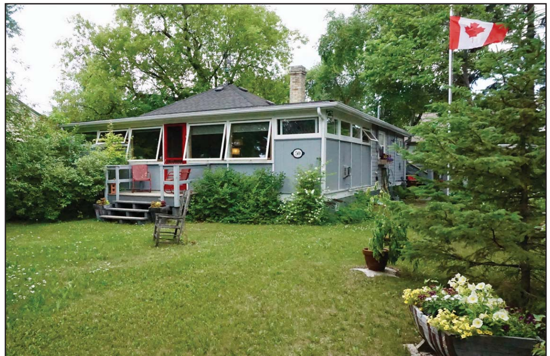
The Thorson Cottage, built in 1918 and restored by Andy and Cindy Blicq, at 50 Fourth Avenue, Gimli.
