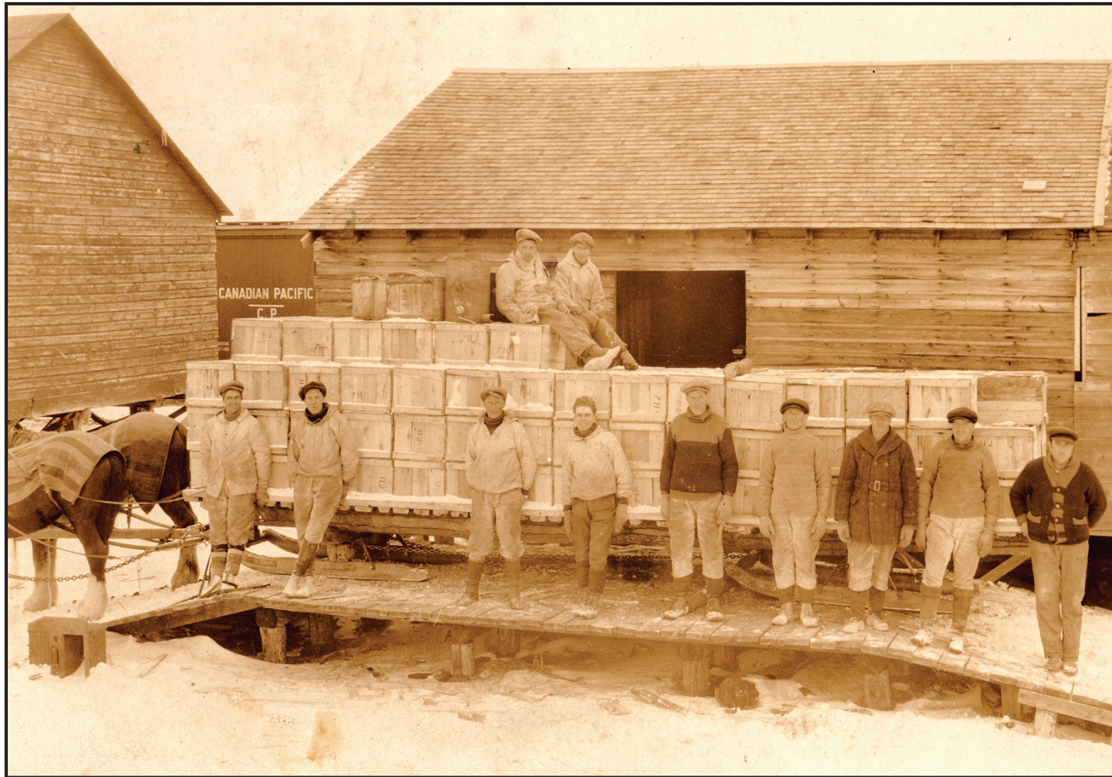
Unloading frozen fish at Gimli, circa 1914. In the early days, advances in the fishing industry improved life in the Icelandic communities along the lake. The work provided badly-needed income. There were jobs building boats and wooden crates to carry the catch, and employment on the freighters and in the administration of the fish companies. By 1907, 5,000 people were employed in the fishery. (NIHM: Grund Stevens Coll.)
