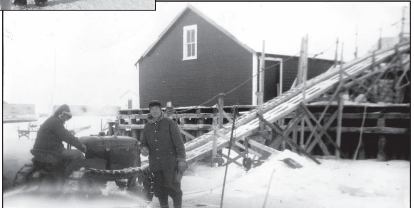
Above: A conveyor belt mechanism powered initially by horses and later by a tractor elevated ice blocks into the insulated storage house. In the weeks and months after, ice was scraped off the blocks and placed in wooden crates along with the fish. These crates were then hauled by wagon to the train station, where they were shipped to market. ( GSM: 686. )
