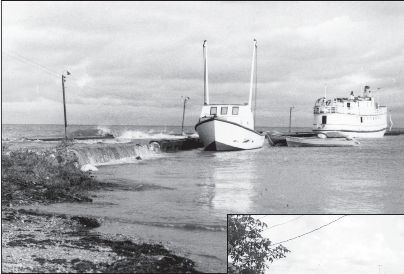
Above: The Gimli pier under water in September, 1966. (GSM: 112.)
