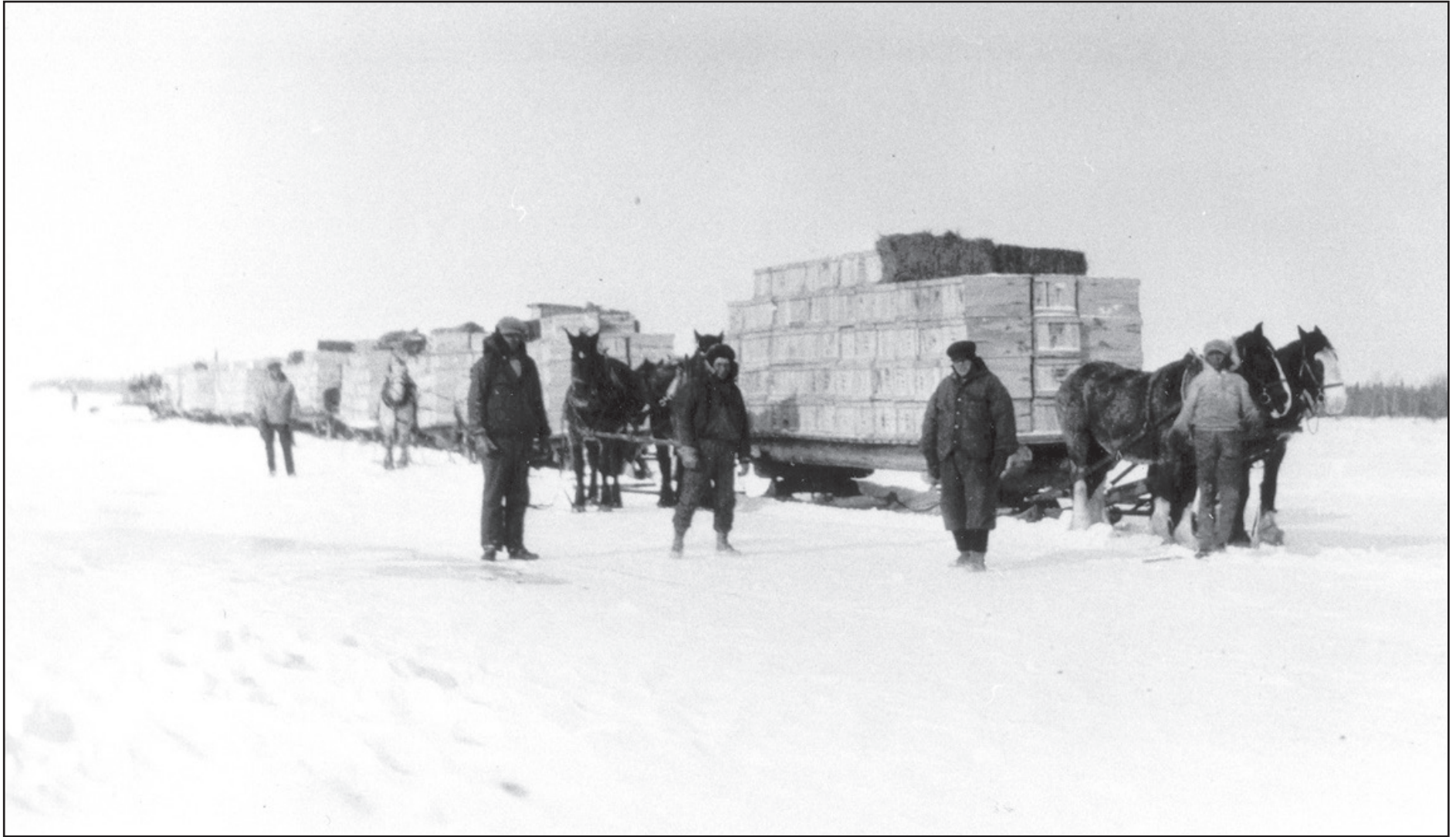
Freighters on Lake Winnipeg, circa 1930s. Two or three teams of horses were normally used, pulling between 8 and 12 sleighs at a time. Each sleigh could shoulder 150 boxes of fish, weighing a total of 7000 kilograms. The train also contained a caboose where the men ate and slept. Conditions were efficient, but primitive. According to Robert Kristjanson, who has spent 70 years fishing on the lake, a tent folded open to make a shelter. The horses were kept on the outside. In the middle there was an area heated by woodstoves that housed a kitchen and bunks for the men. Kristjanson recalls lying in his bunk at night, listening to the horses " chewing and farting. " (Nicholson, 2007:31 and AofM: New Iceland Coll. )
