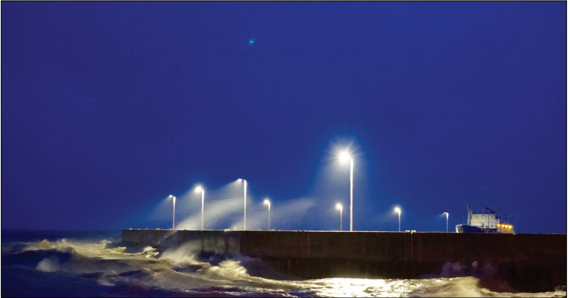
Stormy waters buffeting the Gimli pier. Fall gales on the lake are legendary. In this photograph taken at dusk in November, 2016, waves driven by a strong north wind send plumes of spray over the concrete breakwater. Improvements and upgrades to the harbour in recent decades have made it a safe place for both pleasure and working vessels. Rock breakwaters have been added. Entrance to the harbour is made through a relatively narrow opening to the southeast. (Andy Blicq Photo.)
