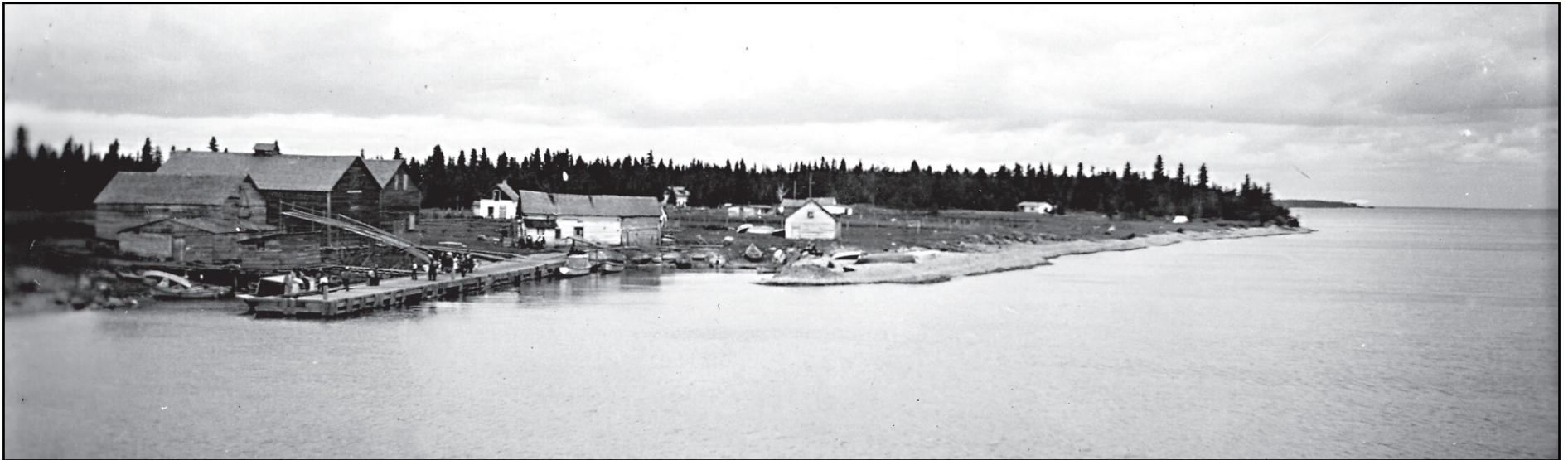
Above: The Snake Island Fish Station in 1934. Fishers lived and worked for weeks and months at these remote stations. In the beginning, camp buildings were constructed of logs. The roofs were made with saplings and hay. The log walls were chinked with clay and in winter, some enterprising crews covered the outer walls with water which quickly turned to ice making a nearly airtight barrier. The larger camps had a bunkhouse and a cookhouse. A cook prepared hearty meals for the crews who worked hard all day in often challenging weather. Down by the waterline, there was often a building for cleaning fish and another for storing ice. (AofM: Loudon Coll. #649.)
