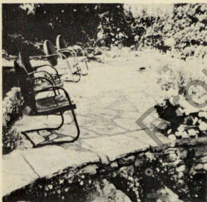
Tyndall stone, as well as precast concrete, slabs are also suited for stepping stones in the lawn or across a planting area. The spacing is important. For convenient walking, the centre of the slabs should be 25 inches apart. Each individual slab should be at least 2.5 square feet in size and may be laid in sand or directly into the ground.
