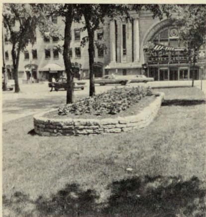
Most important for all wall or planter construction is the placing of perfectly horizontal layers. On this sloping area, three layers of stone are visible on the right side of the planter, while four layers can be seen on the left side.
