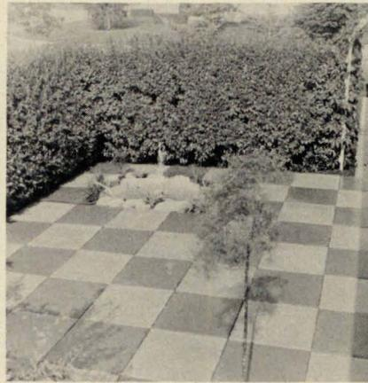
Precast concrete blocks have been generally accepted as durable material for patio and walk construction. Here, 2' x 2' slabs are forming a patio in checker-board fashion by the use of red and natural colored blocks.
