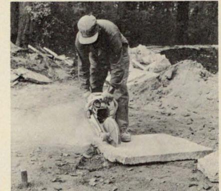
If narrow joints are desired, Tyndall stone may be cut on the construction site and fitted closely together
