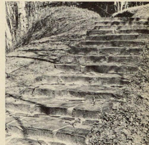
A rustic but safe stairway, blending well into the landscape. Split granite, laid in concrete, has been used with steps protruding above the face of the slope.
