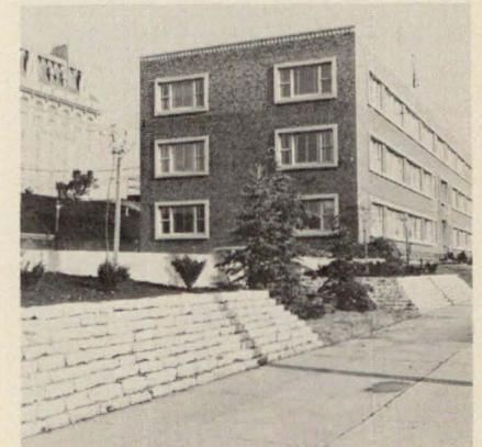
A well built, stable retaining wall of Stony Mountain limestone. An interesting effect is achieved by using a setback of 3" for each layer.
