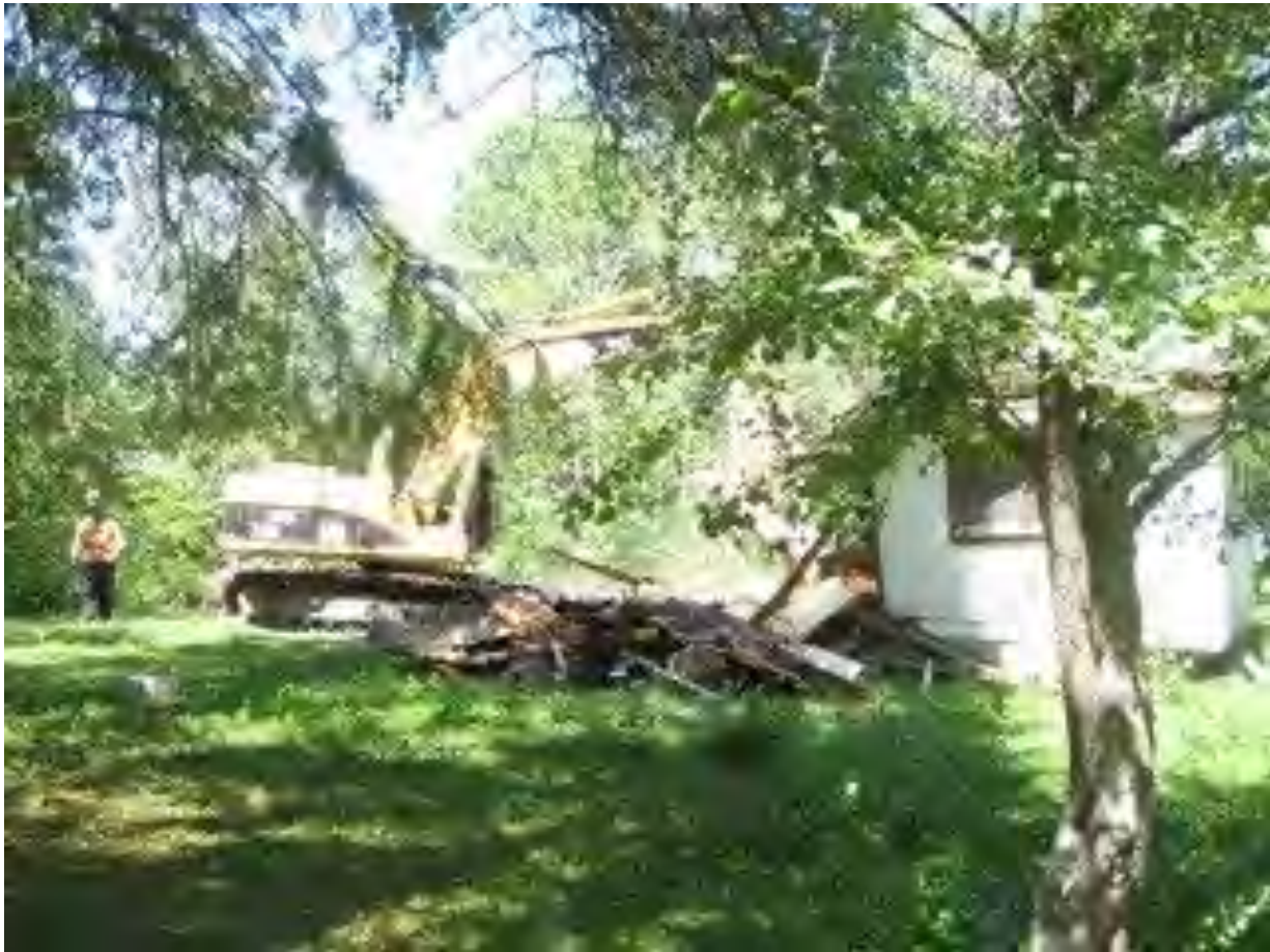
Demolition of original cottage 2010
