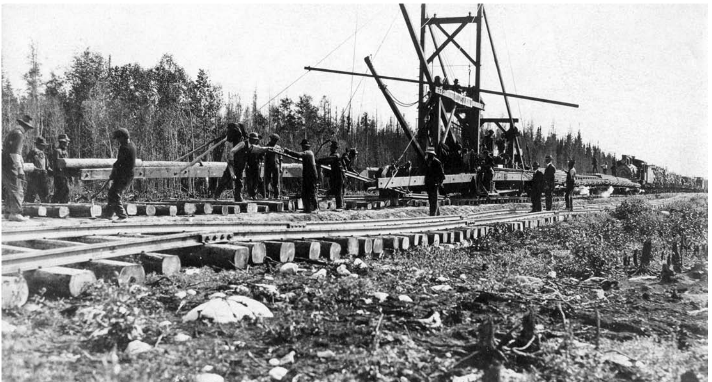
The Hudson Bay Railway under construction, circa 1920.
