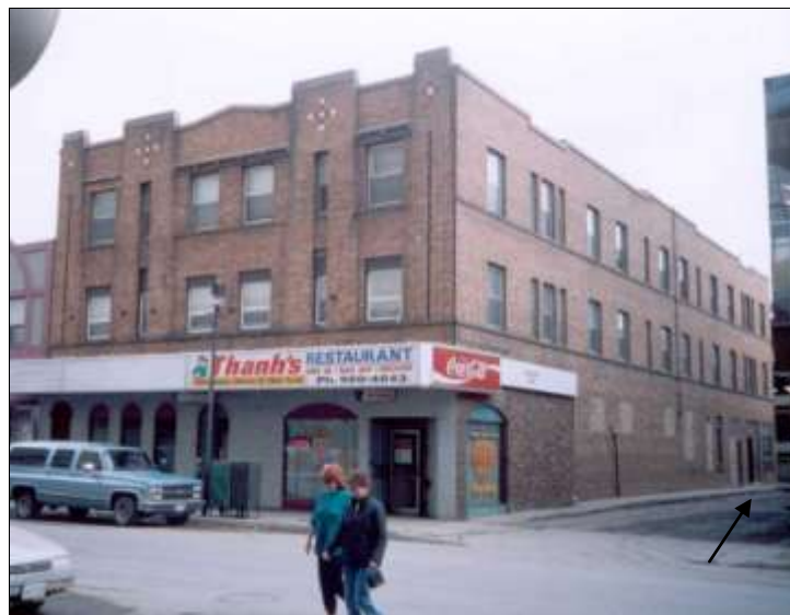
Davin Building, 1765-69 Hamilton Street (faced with T-P Moka brick made at the Claybank Brick Plant)
